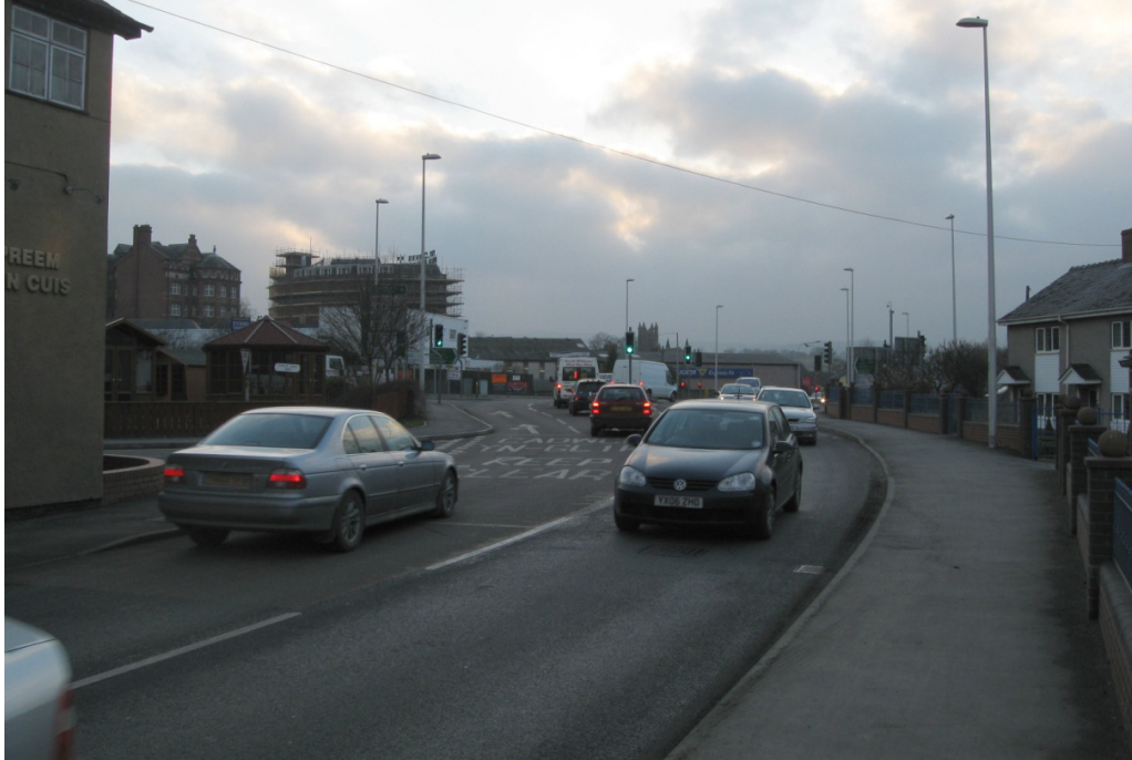
Photograph 3.1: Showing the poor straight through alignment from Pool Road.
